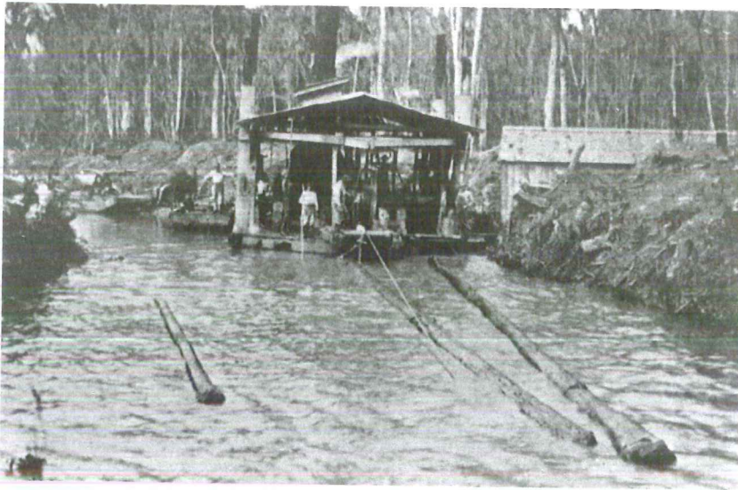
FIGURE 4.15 A two-drum pull boat working in a canal that was cut into a cypress swamp in Louisiana (date unknown). (From Williams 1989.)
